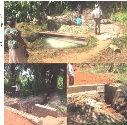
A New Protected Water Source: Before & After
