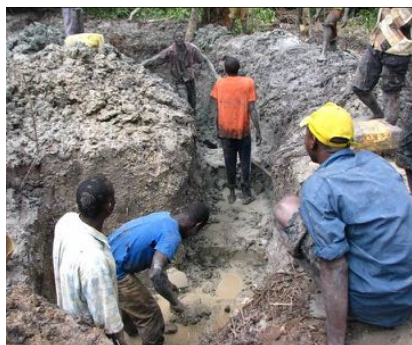
Omni Med staff working with local villagers, constructing a ditch that will be filled with sand, clay, and porous rock to filter and clean the water
